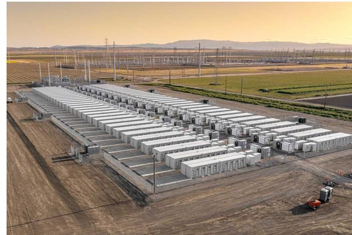
**Utility-scale BESS to the California Independent System Operator, with 548 MWh capacity, supporting 26,000 homes**
