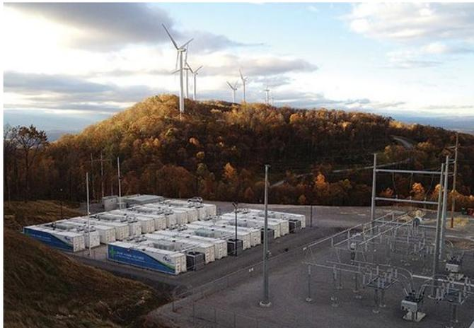
**BESS installation can smooth out variability in the adjacent wind farm, supporting 1GW into the Grid over 4-6 hours**
